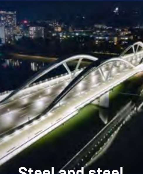
Steel and steel plant construction 10.1 %
