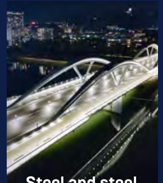
Steel and steel plant construction 8.6 %
